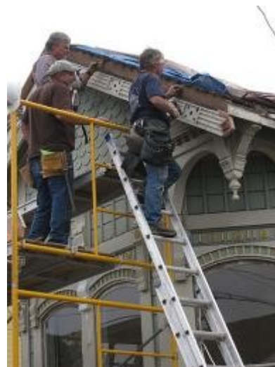
Above, members of the California Conservation Corps remove layers of old shingles, exposing the original skip sheathing of the roof. Below, Wes Marshall and Mike Coop, students in the Field School, along with instructor Bob Felter, repair the front gable.
