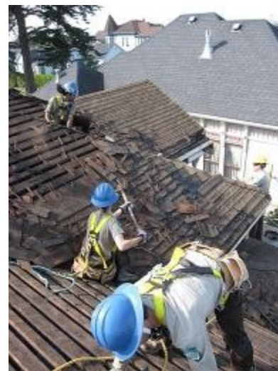
Above, members of the California Conservation Corps remove layers of old shingles, exposing the original skip sheathing of the roof. Below, Wes Marshall and Mike Coop, students in the Field School, along with instructor Bob Felter, repair the front gable.
