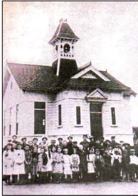
The second Worthington School, a striking Stick-Eastlake, was built in 1893, replaced in the mid-1910s, then moved and turned into a private home that still stands today.
