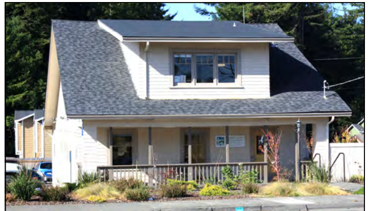
In 1916, the McCabe family moved into this Craftsman on Myrtle Avenue. Today it serves Hospice of Humboldt.
