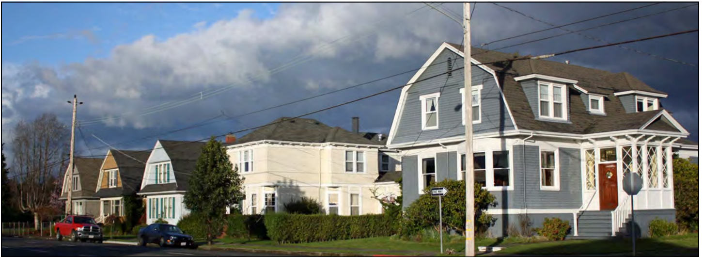
These houses on H Street were built in the early 1900s for noted contractor Harris Mercer, founder of the Mercer-Fraser Co.
