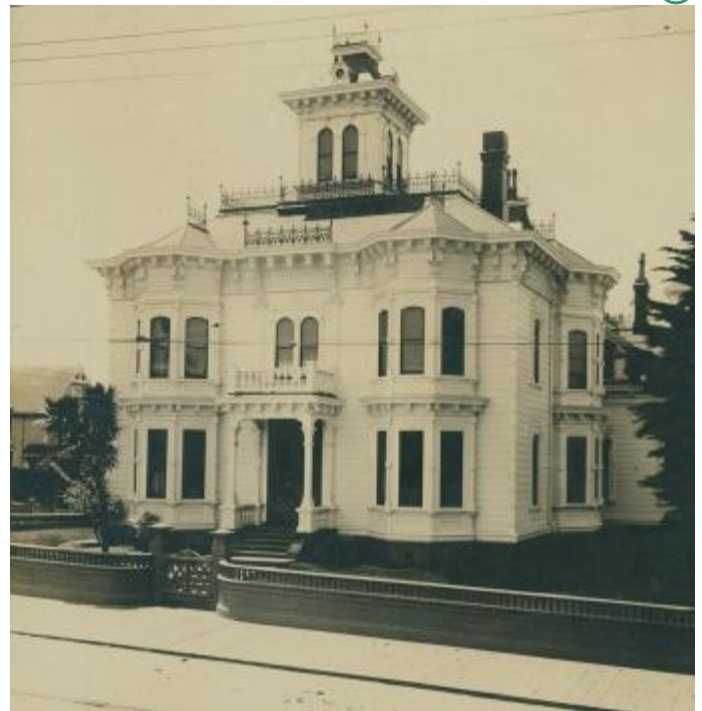
David Evans home Main elevation from E Street
